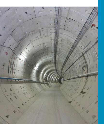
Segment lining offers distinct advantages and challenges when compared to pipe jacking. Unlike pipe jacking, segment lining is not restricted by length and diameter, making it the preferred choice for longer and larger-scale tunnel projects and more challenging environmental requirements. This flexibility is one of its key advantages, allowing for the construction of extensive tunnels without the constraints associated with other methods.
