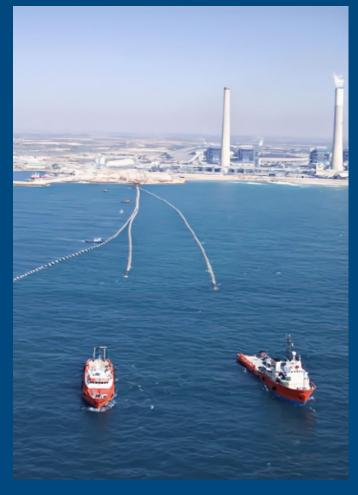
**IDE Technologies** is executing an intake and discharge project for the Aconcagua desalination plant in Chile. By employing two jetties, IDE overcame the region's challenging coastal conditions, which limit the working season, and provided stable platforms for the excavation and trenching operations required for the intake and discharge pipelines.
